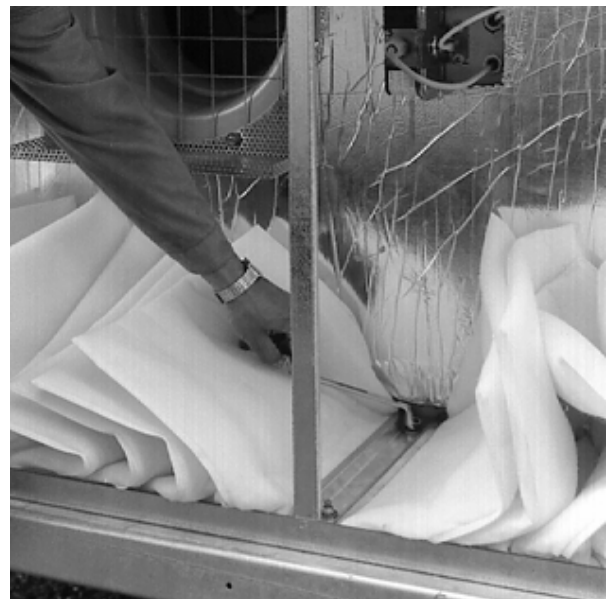
Fig. 11c Removing the filter support (Two hex. nuts, wrench size 14)
